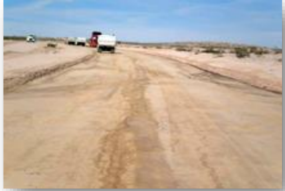
Completed NATURALPAVE System
