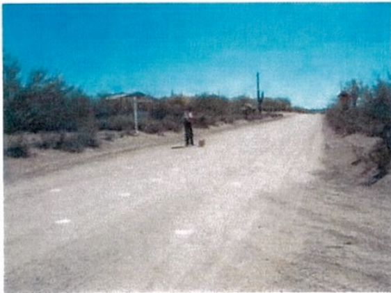
Site 3 Looking East
