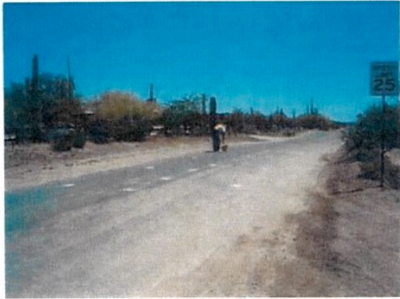
Site 5 Looking East
