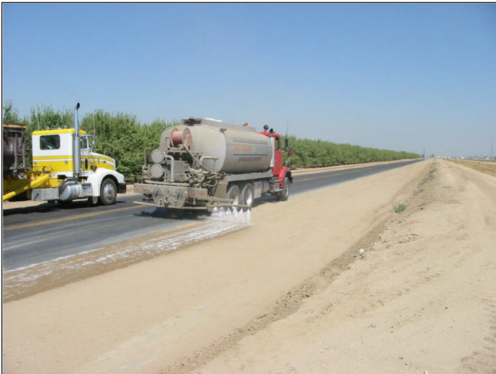
Photo 2 Soil Sement – First Coat Looking North on Allen between Kratzmeyer and Snow
