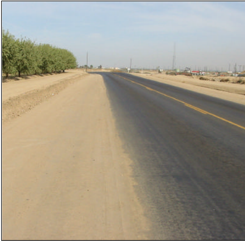
Photo 4 Demarcation Between Untreated Soil and Soil Sement® A Vehicle Used the Shoulder and Performed a Hard Acceleration
