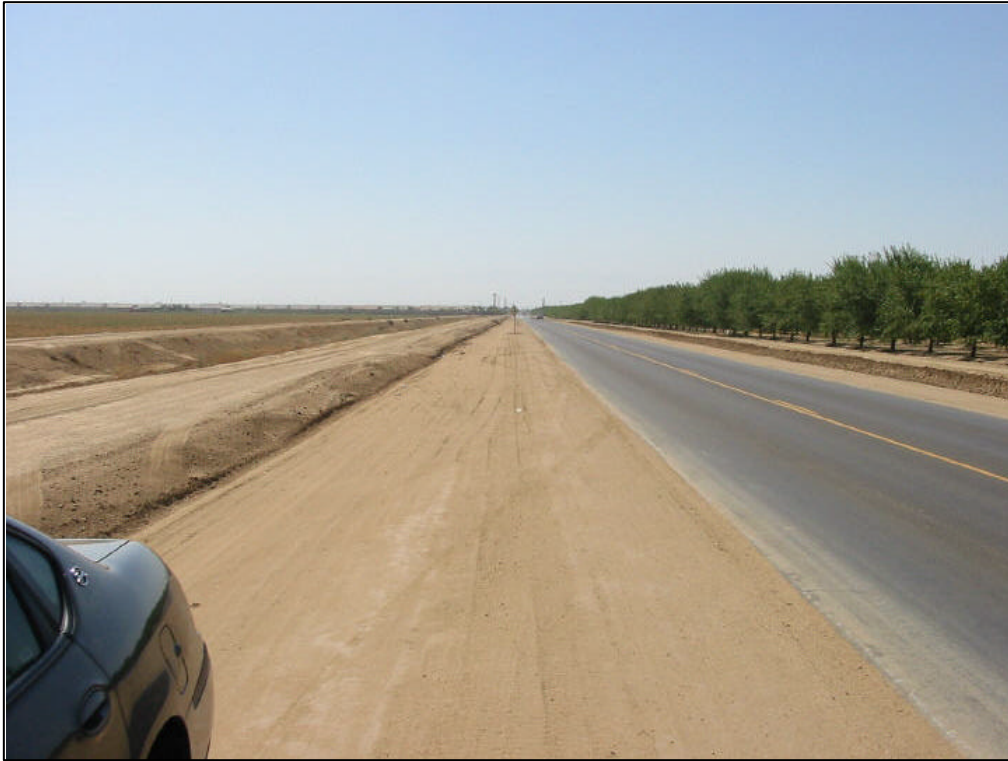
Photo 2 Soil Sement – First Coat Looking North on Allen between Kratzmeyer and Snow
