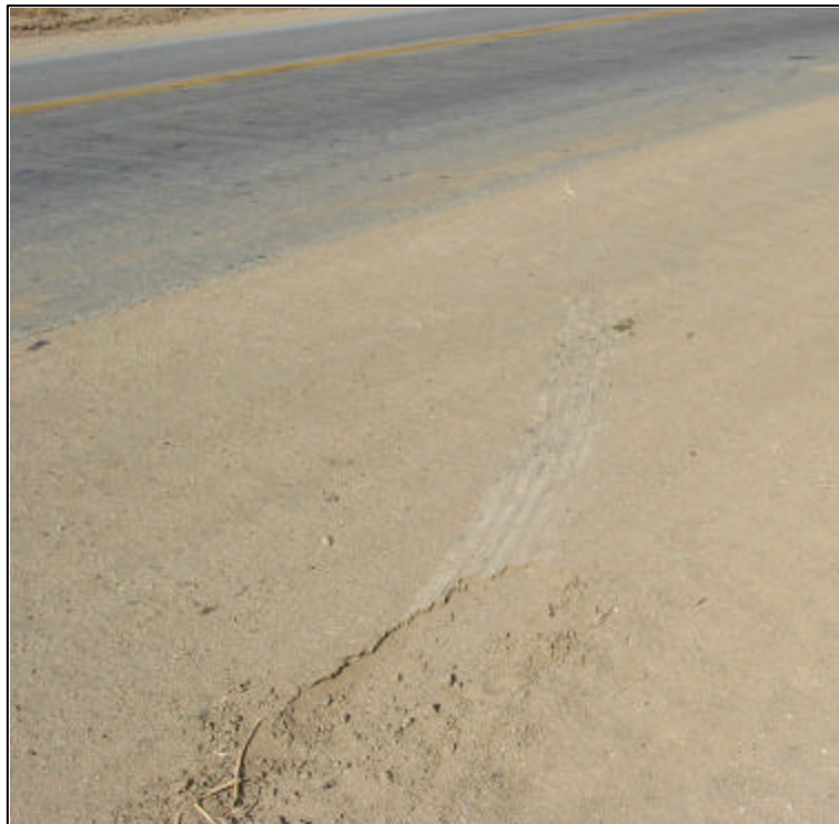
Photo 4 Demarcation Between Untreated Soil and Soil Sement® A Vehicle Used the Shoulder and Performed a Hard Acceleration
