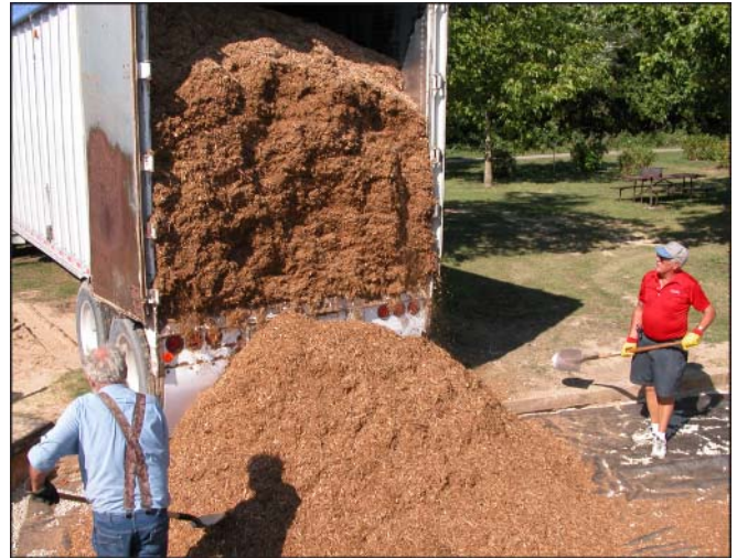
Figure 5—Application of engineered wood fiber (EWF).
