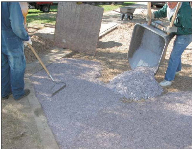
Figure 7—Leveling and compaction of binder–EWF mixture.
