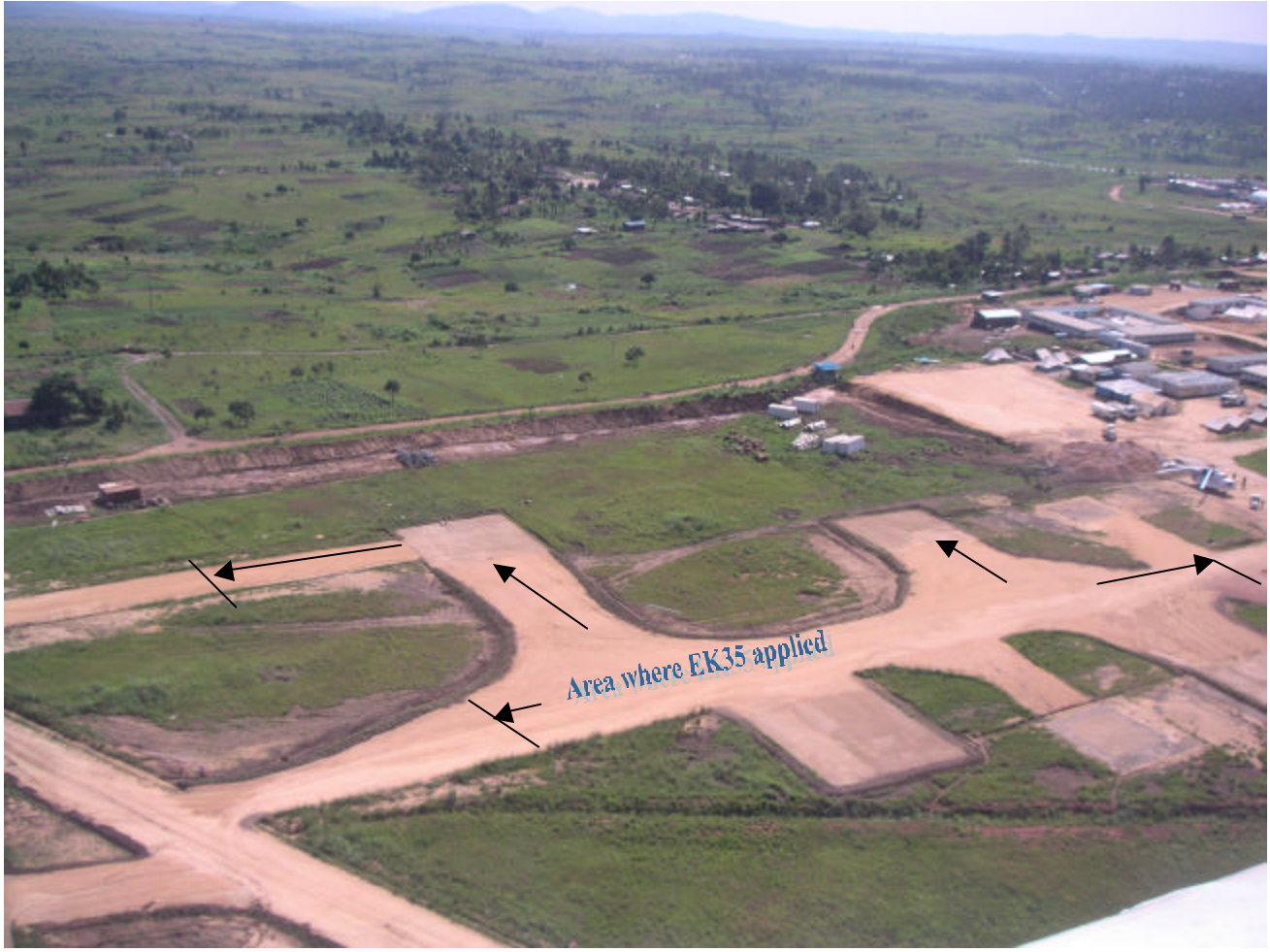
Helipads at Bunia airport site.
