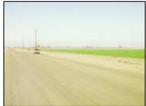
SOIL-SEMENT® stabilized dust-free shoulder
