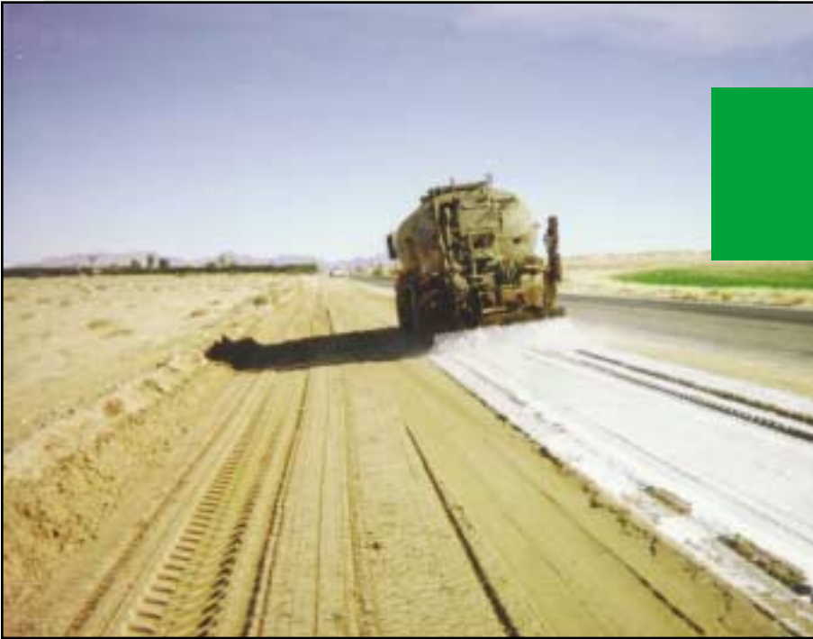
Topical application of SOIL-SEMENT® onto shoulder
