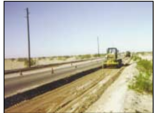
Blade mixing SOIL-SEMENT® into unpaved shoulder
