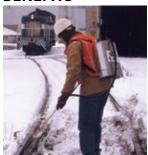
Ice Free Switch is an anti-icing agent used to prevent switch freezing from falling and blowing snow and icing conditions. When applied to switch points, plates and rail prior to snow or ice storms, it will remain in place to activate when needed to melt falling and blowing snow and prevent switches from freezing.
