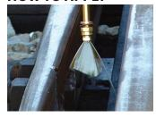
Once the switch is clean, brush, pour, or spray Glidex track switch agent onto the appropriate components. Spraying is usually the preferred method as it is the easiest and quickest. Put a light even coating on the surfaces to be treated. A typical application will require about 8 to 10 ounces of product. Glidex track switch agent can be applied to a wet switch without impairing product performance.
