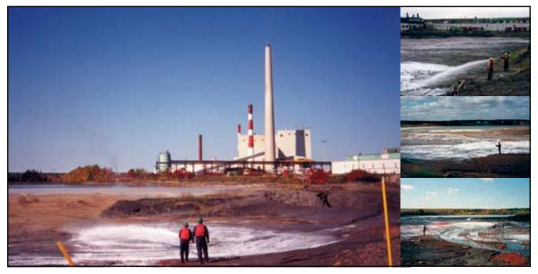
Soil-Sement® has the unique ability to eliminate dust and airborne particles because it chemically bonds and seals the surface to prevent wind from lifting fines and creating dust.
