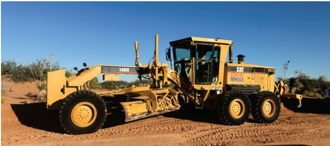
Figure 28. Motor grader used for test section construction.
