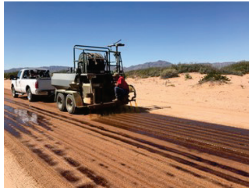
(b) Surface after spraying Item 4.
