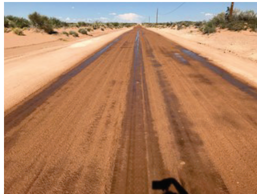
(b) Surface after spraying Item 2.
