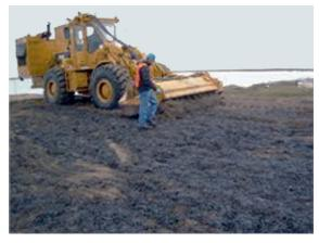
Discrete SF2 fibers, lightweight, with high-tensile strength, are combined with a Midwest Synthetic Organic fluid and then compacted to create a surface that can increase CBR by up to 400%.
